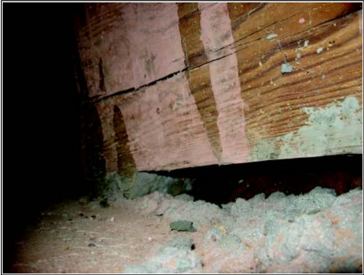
Figure 26. Gunstock post in parlor
