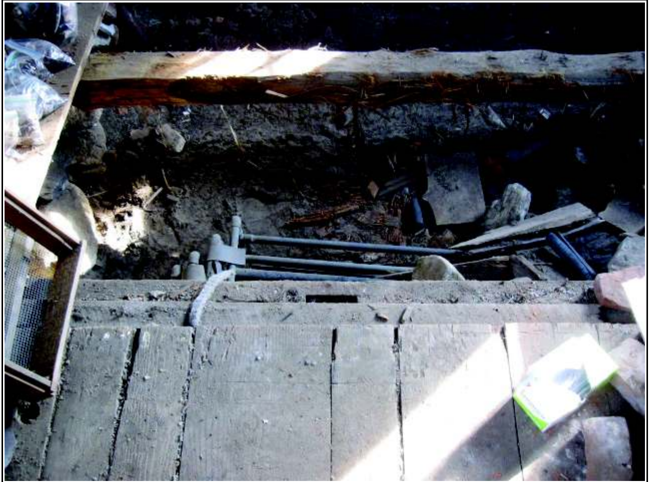
Figure 23. Bark covered floor joists in the North Ell
