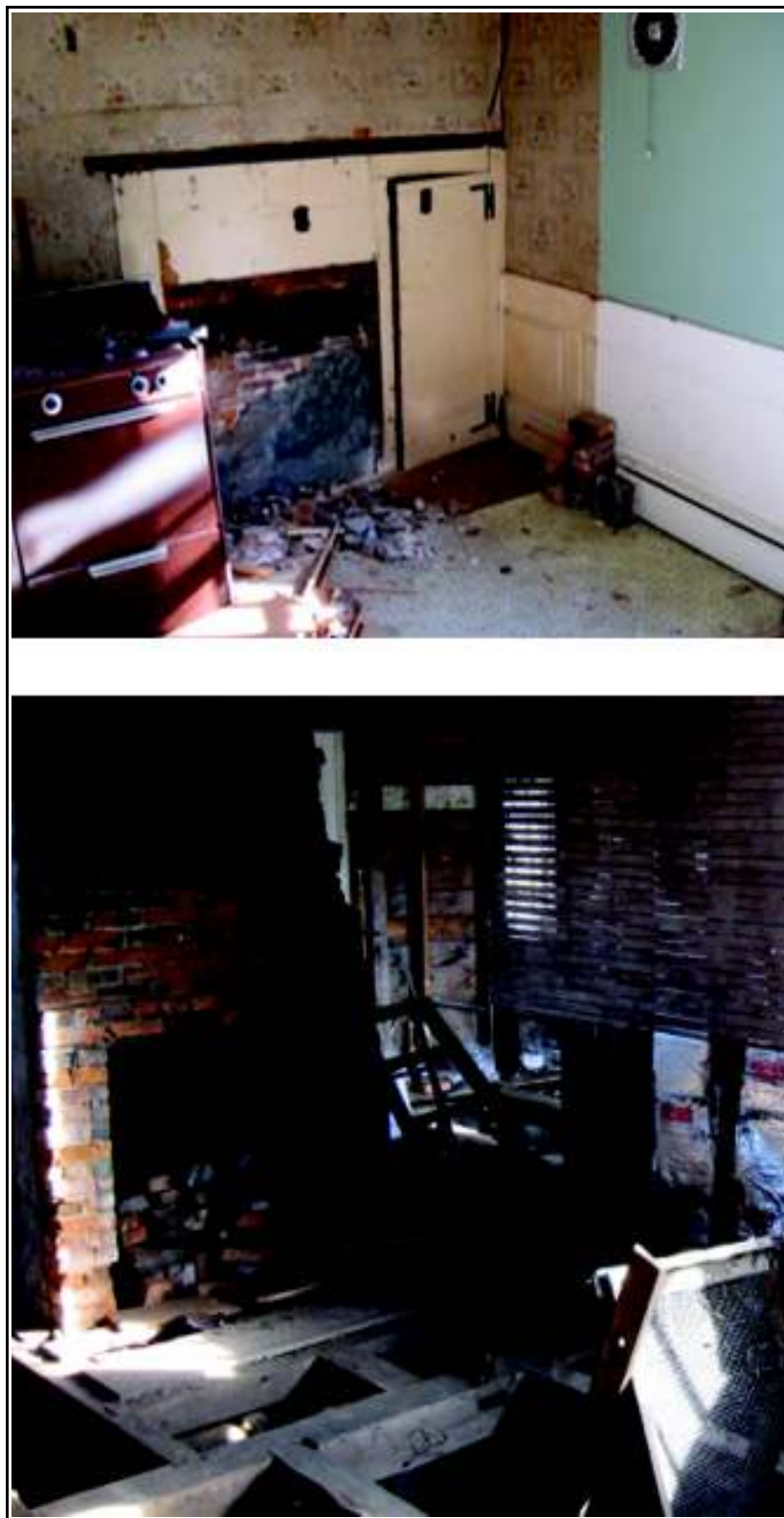
Figure 22. Center Ell hearth before and after renovation stripping
