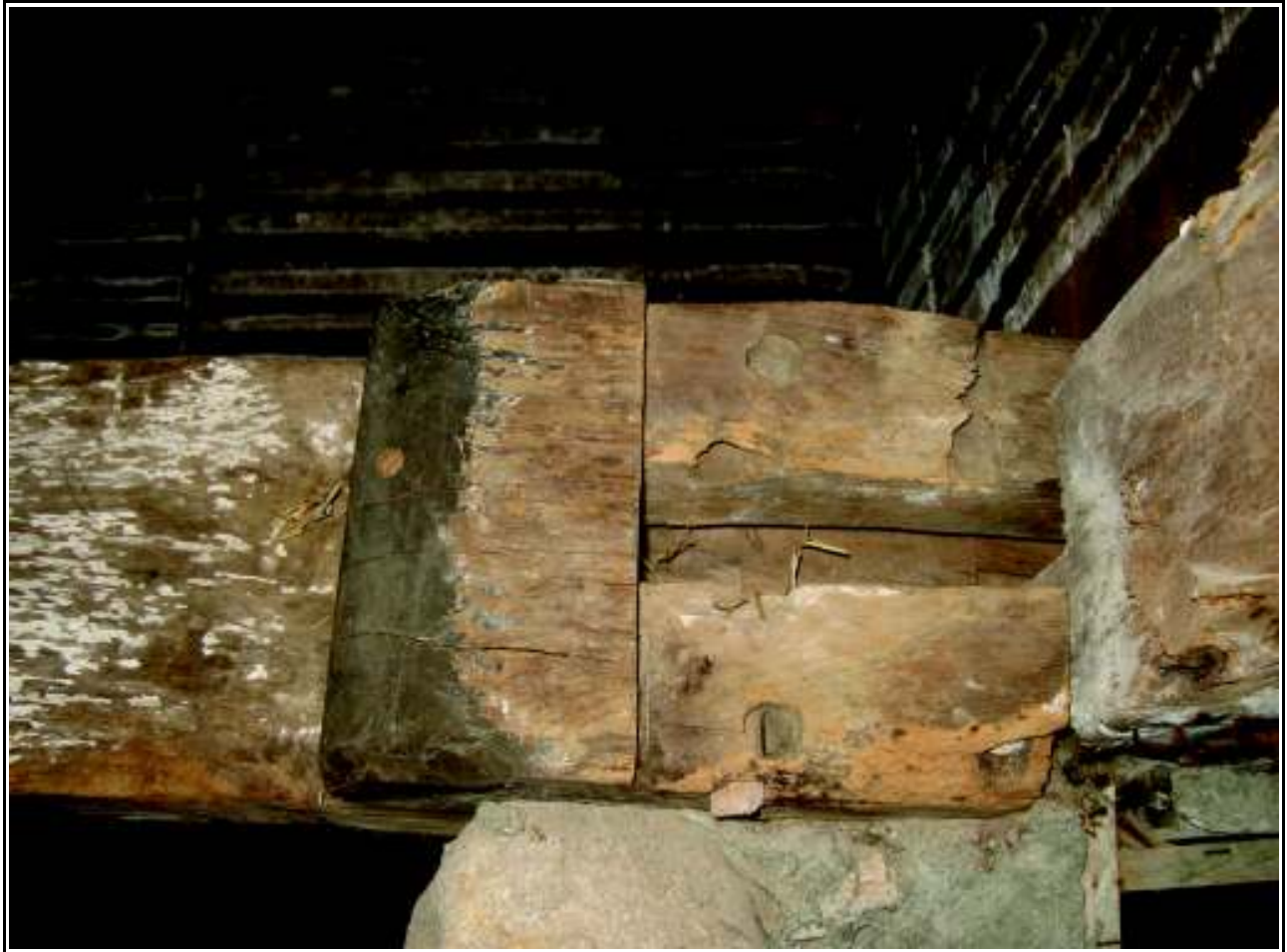
Figure 29. "Ship's Timber" in former bathroom used as joist
